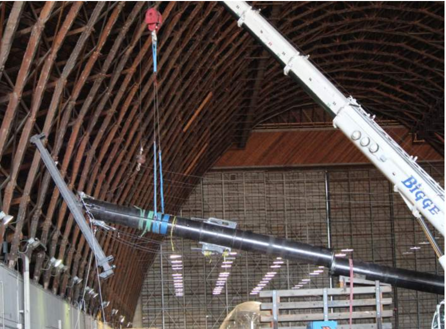
Hoisting of temporary shore segment
