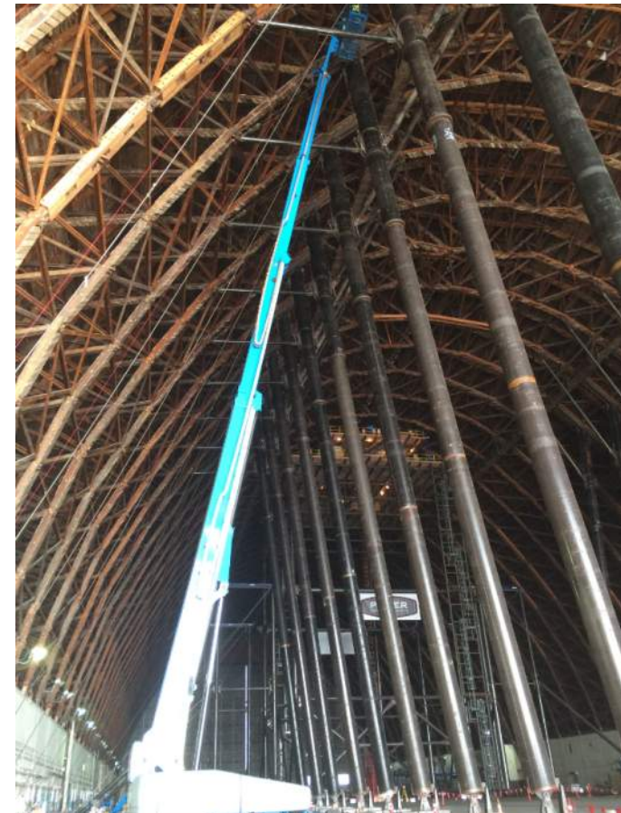
Boom lift used for visual observations
