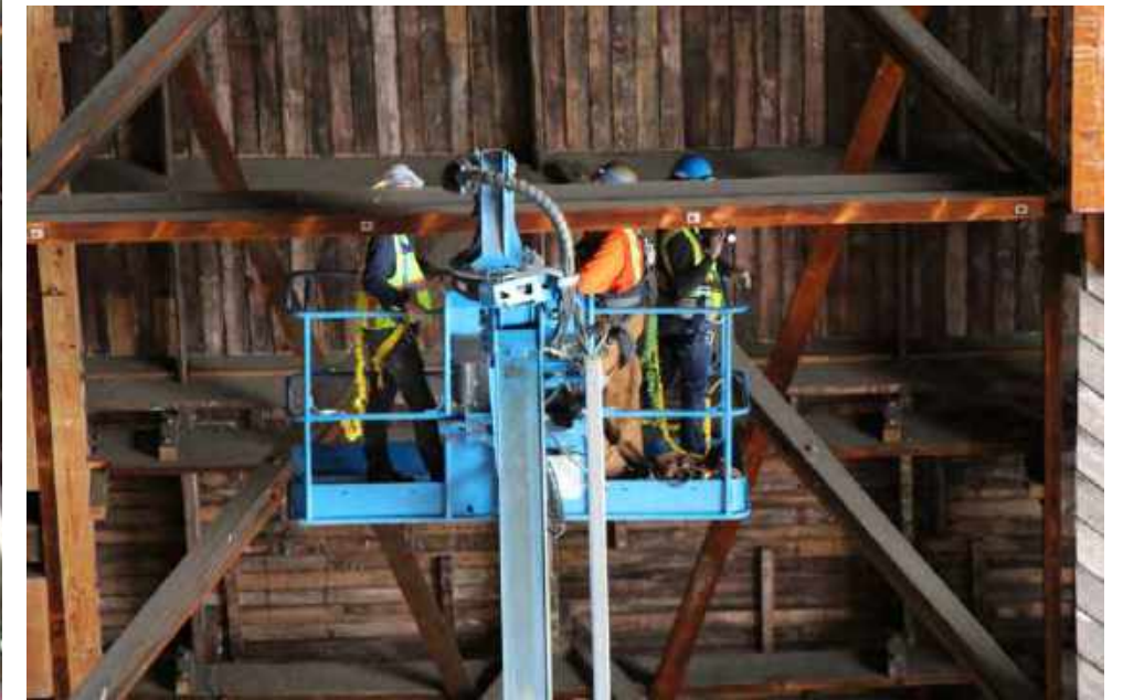
KPFF condition assessment crew
