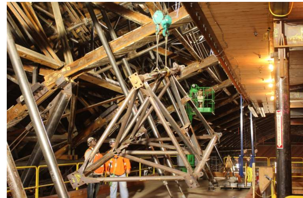
Hoisting exoskeleton segment into place
