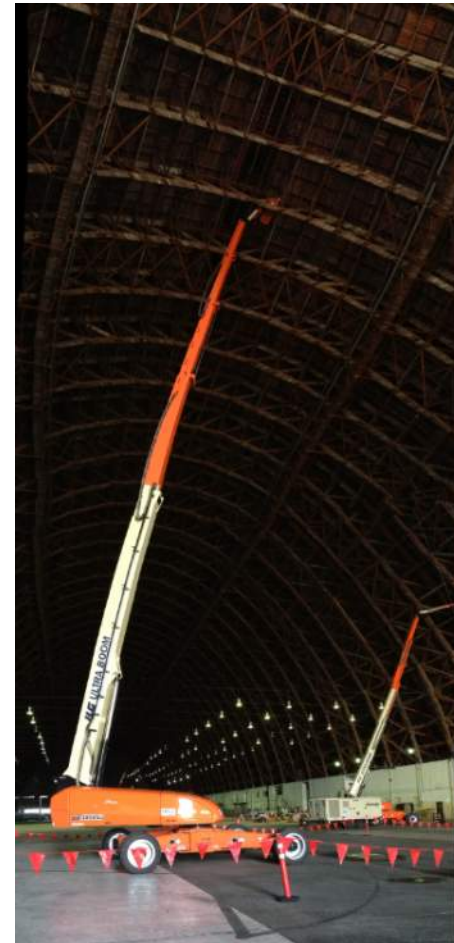
Boom lift used for visual observations
