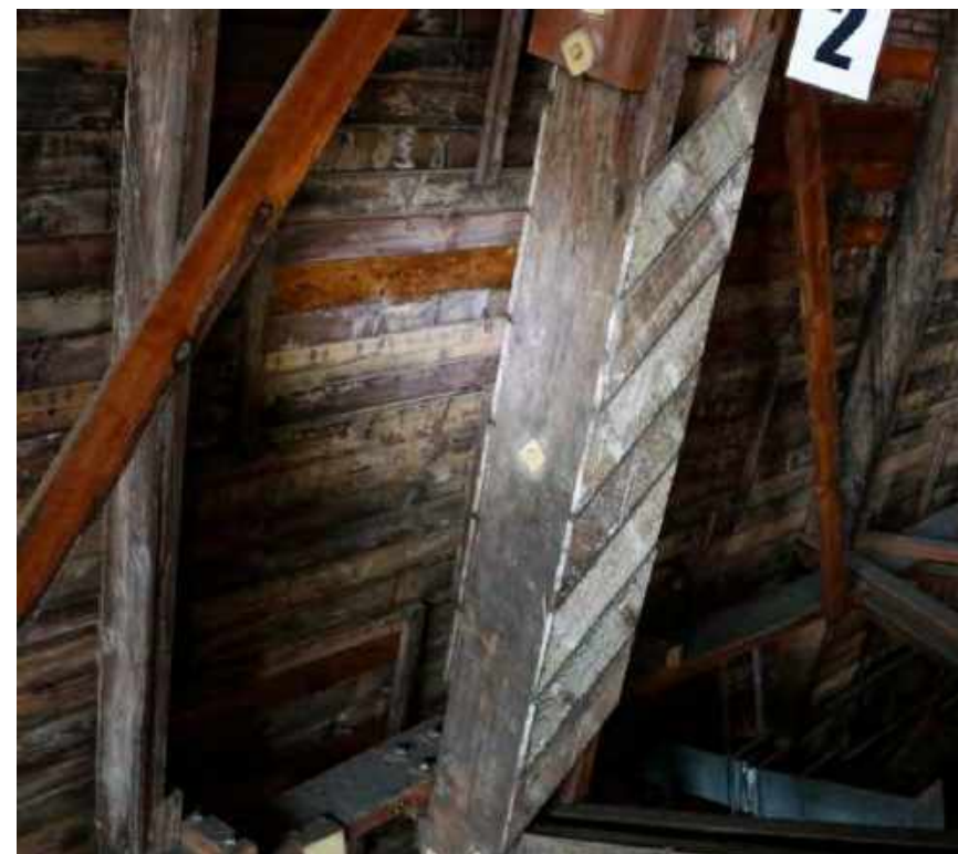
Typical chord member with battens
