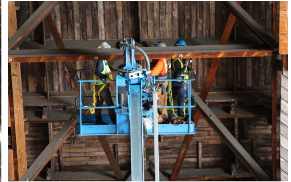
KPFF condition assessment crew
