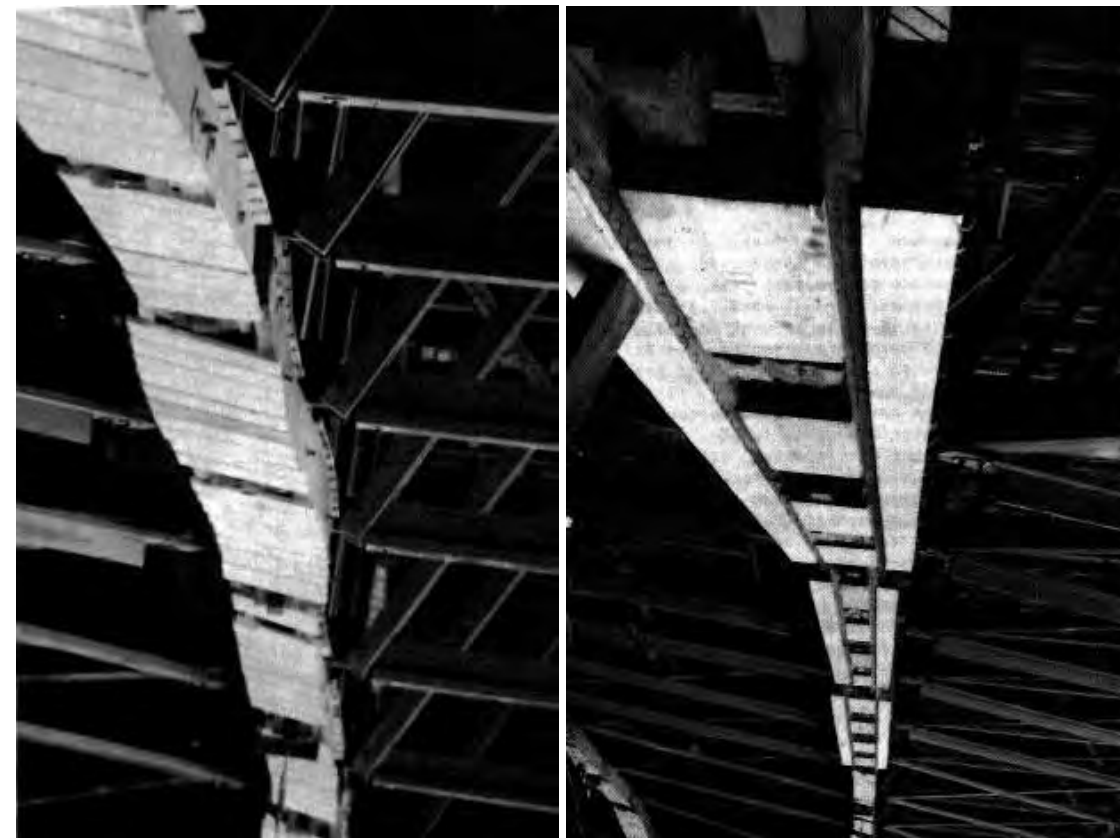
Buckled chords (left) and glulam strongback repairs (right) - "Restoration of Navy LTA (Lighter than air) Hangars", Donal Neal, 1986
