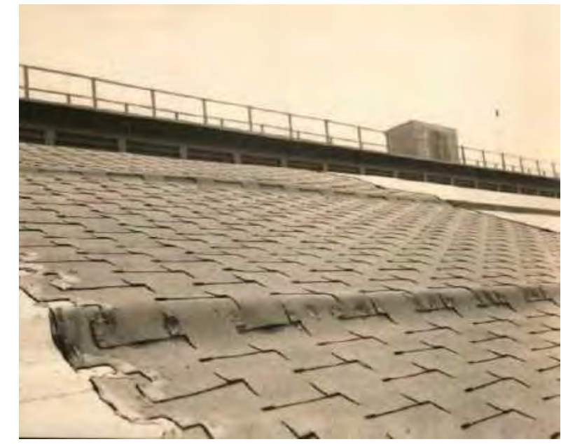
Asphalt shingles documented in 1954 -Seabees Historic Photos
