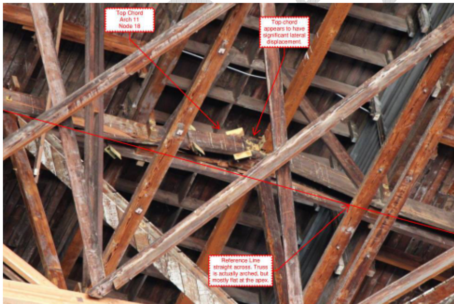
Figure 5. Relative lateral displacement between arch apex and reference line for Hangar 3 single arch.
