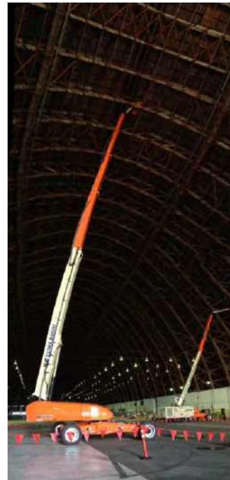
Boom lift used for visual observations
