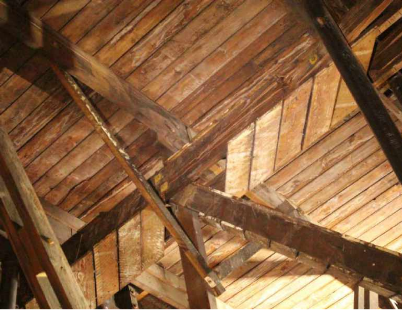
Typical vertical web member with added knee-braces
