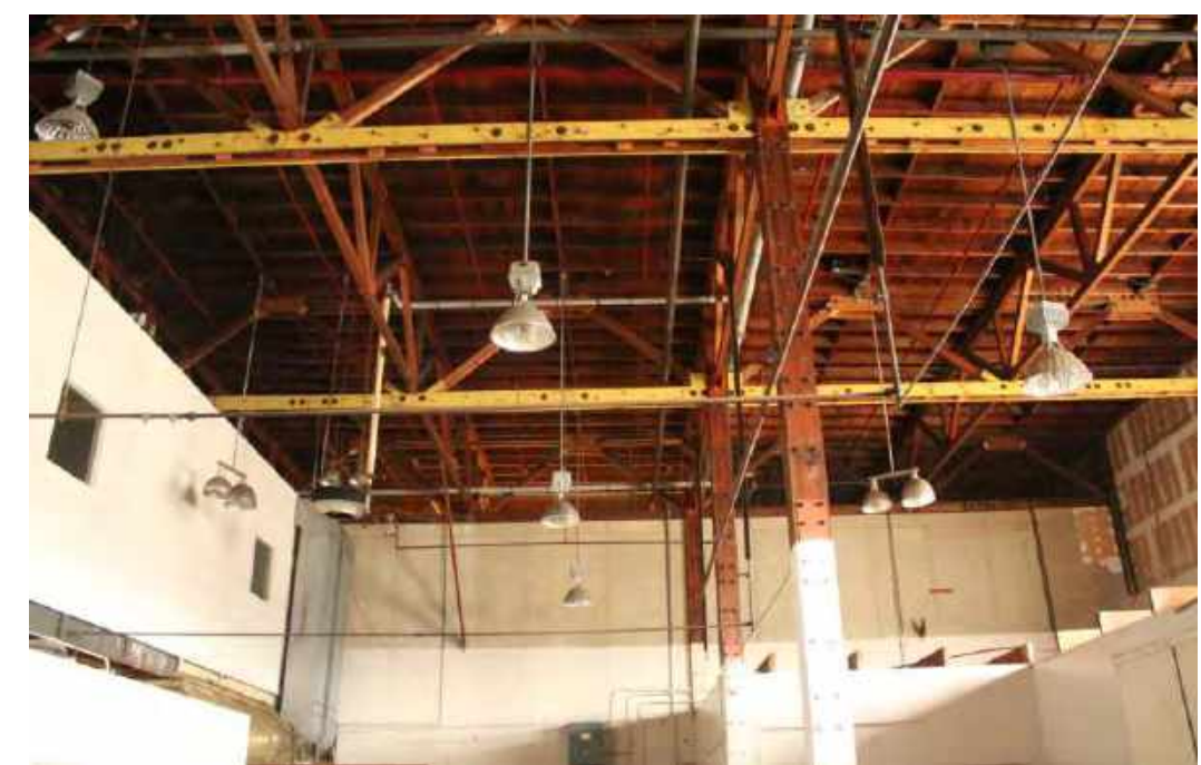
Interior view of Hangar 3 East Shed Annex
