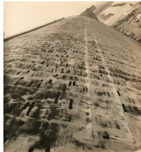
Original roofing system -Seabees Historic Photos
