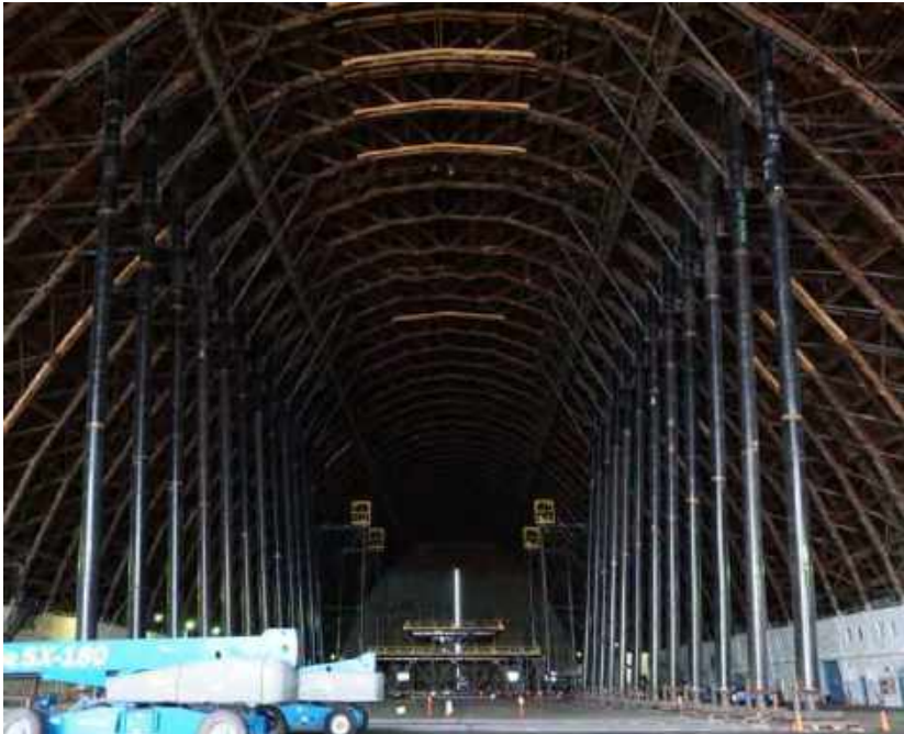
Temporary shores after installation
