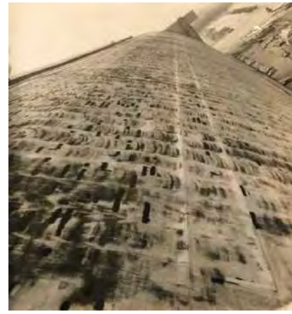
Original roofing system -Seabees Historic Photos
