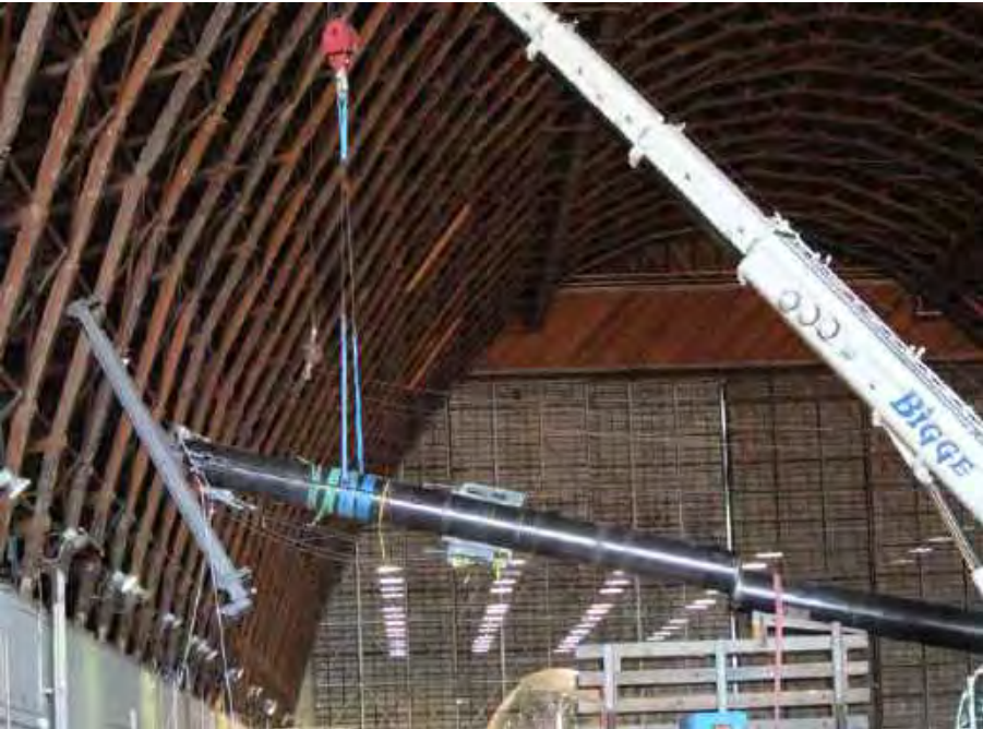
Hoisting of temporary shore segment
