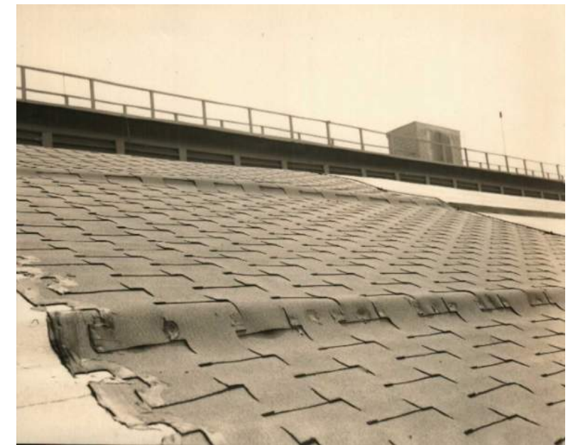
Asphalt shingles documented in 1954 -Seabees Historic Photos
