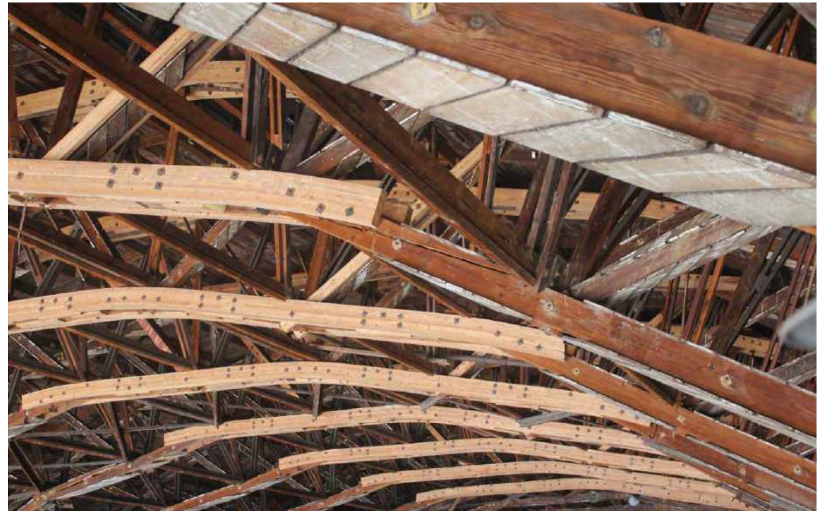
1993 glulam sister repairs to chord members in critical zone
