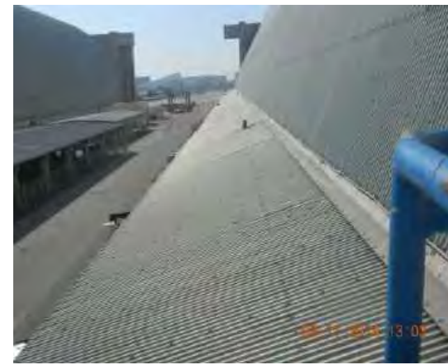
Current aluminum roofing
