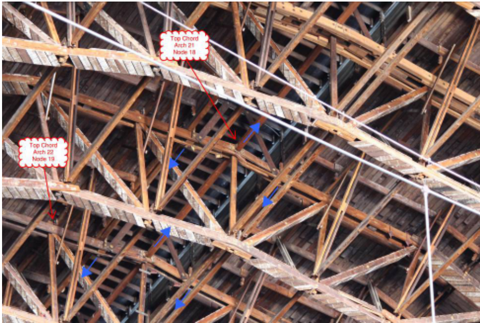
Figure 7. General trend of relative lateral displacement at the arch apex top chord in Hangar 3.
