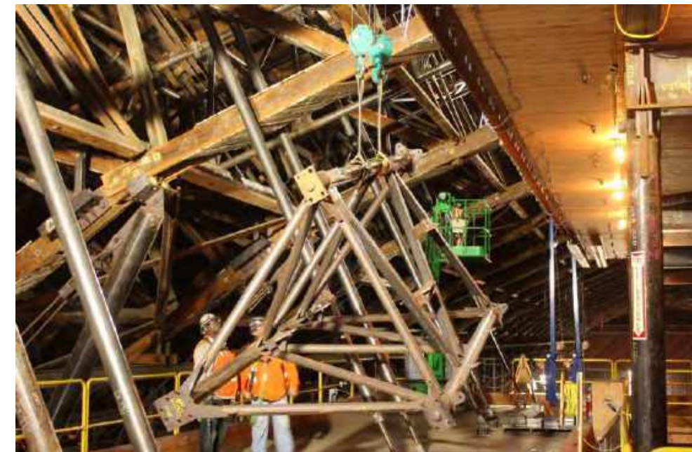
Hoisting exoskeleton segment into place
