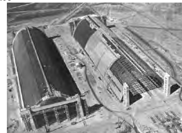
Hangars 2&3 under construction -US Navy Historic Photos
