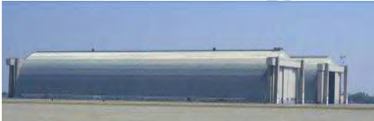
Figure 2. 2013 Hangar 2 (nearest hangar) and Hangar 3.
